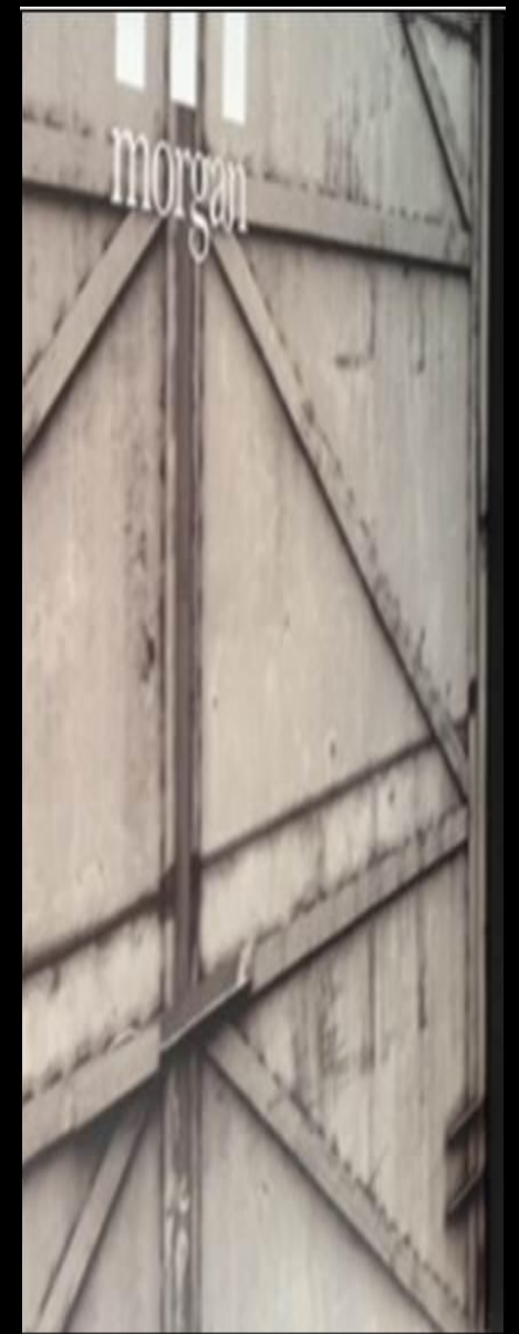
Entry Door to Meeting Rooms
